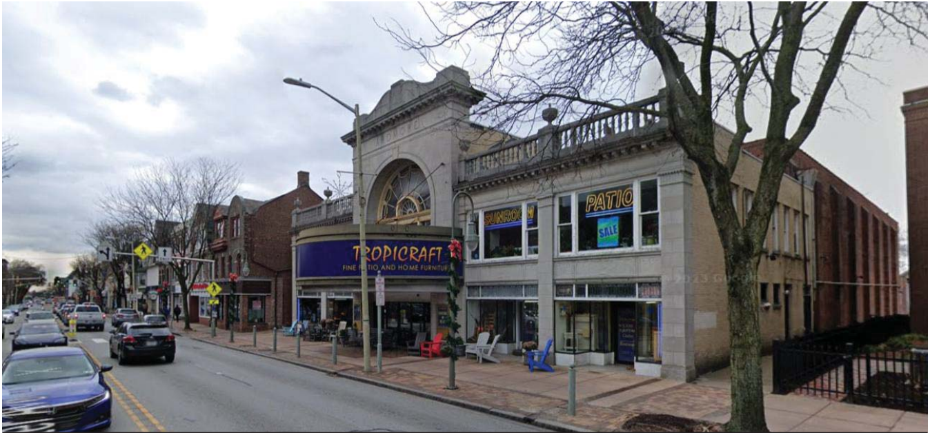
30-38 West Lancaster Avenue – Ardmore Commercial Historic District
