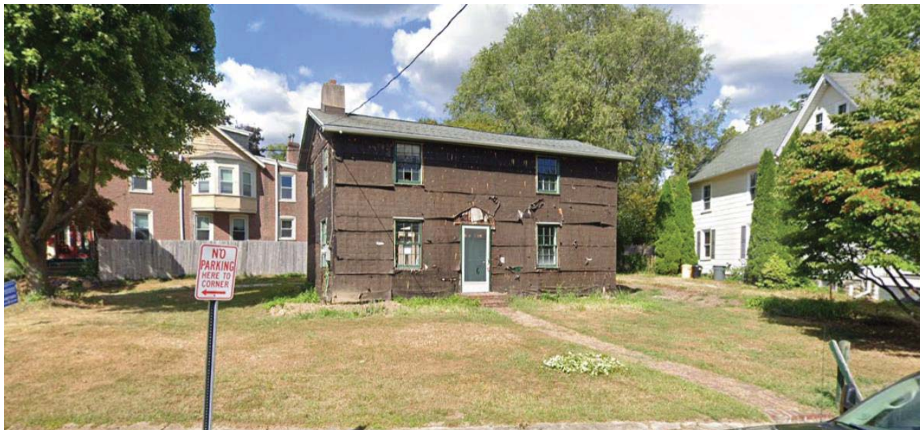
527 Old Lancaster Road, Haverford Station Historic District
