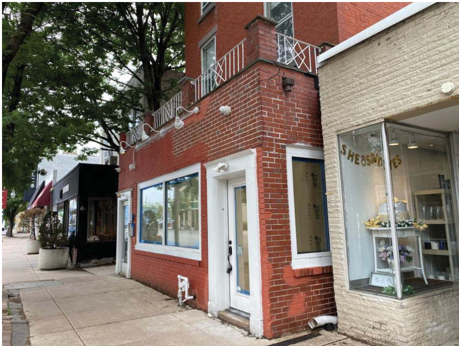
Work was stopped when the unapproved painting work was observed
