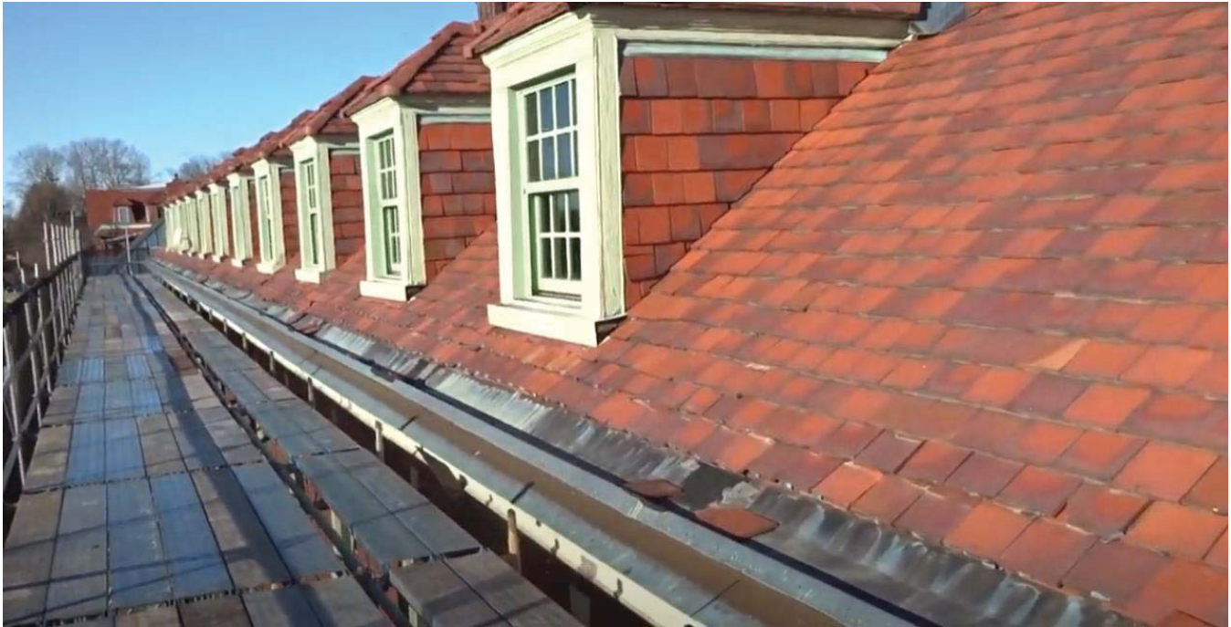
View of Dormers With Tile Roof in Place – Southeast Roof Face
