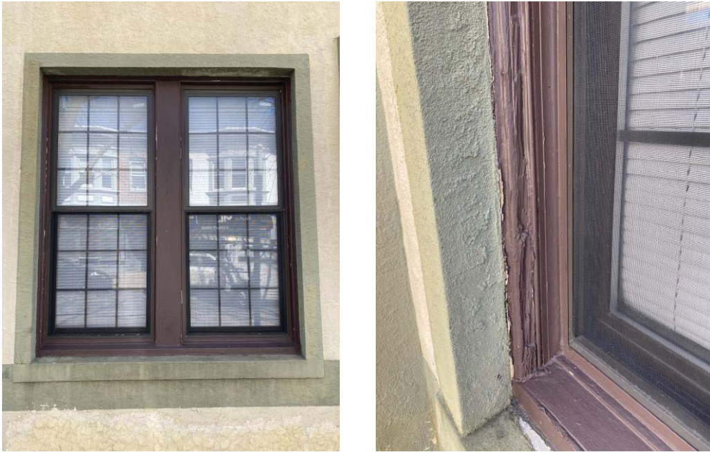
Window trim is in various states of repair/disrepair
